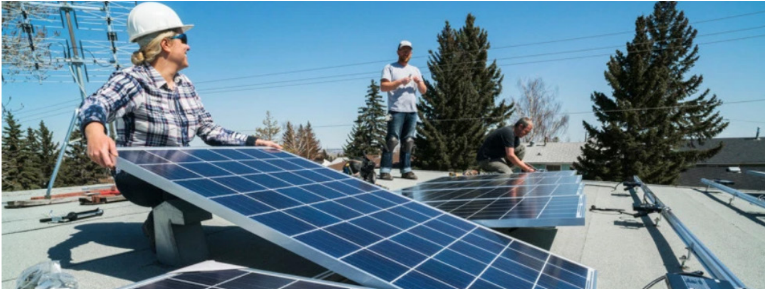
Workers installing solar panels on a residential homes roof.
